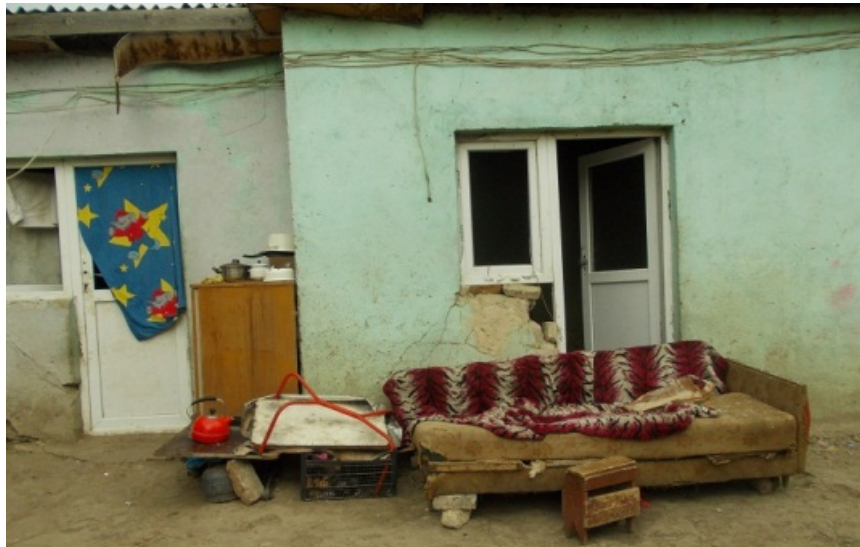
Figure 1: Living Condition in Roma Housing Unit, Samgori District, Tbilisi (Photo Taken by Author) Some 75 Roma individuals occupy a small commune in the Samgori District. Though living quarters are cramped and there is limited access to water and electricity, the families are happier living here than they have been elsewhere as the unit's proximity to the city dump discourages the presence of onlookers, outsiders and harassment by police (personal interview, September 2012).
